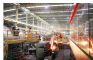
美国连铸连轧生产线 American Southwire Continuous Casting and Rolling Production Line
